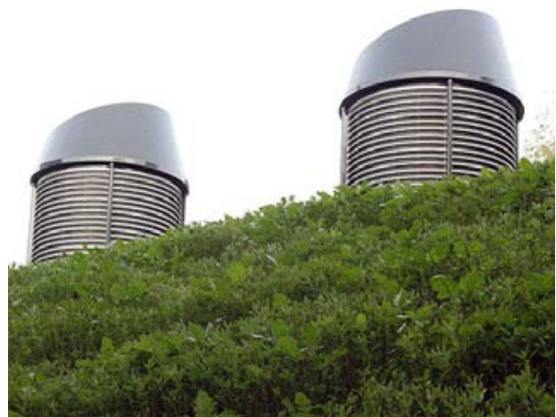
Figure 1. Prefabricated ventilators which utilize the Venturi effect. 3
