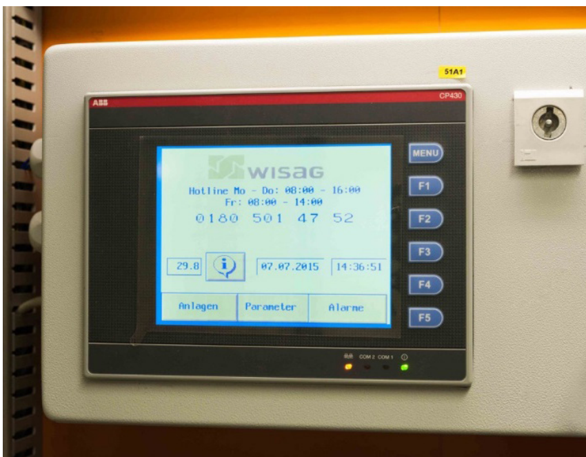
Figure 2. All controls are operated via the touch screen of the CP430 control panel.
