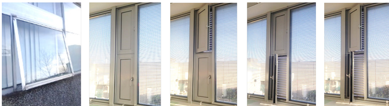
Figure 2. Ventilation system configurations, from left to right: existing building window (CS.01), Retrofit space no ventilation scenario (RS.01), bottom manual louvre only (RS.02), top automated louvre only (RS.03), both louvres opened (RS.04).
