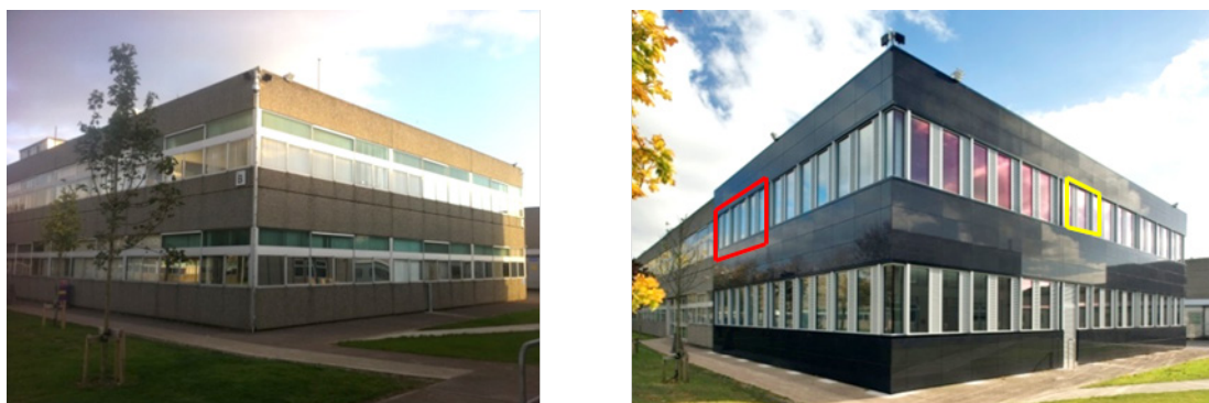
Figure 1. External facades; existing 1974 building (left) and retrofitted zero2020 test-bed building (right) where red indicates the location of the thermal comfort study and yellow indicates the location of the ventilation rate performance experiments.
