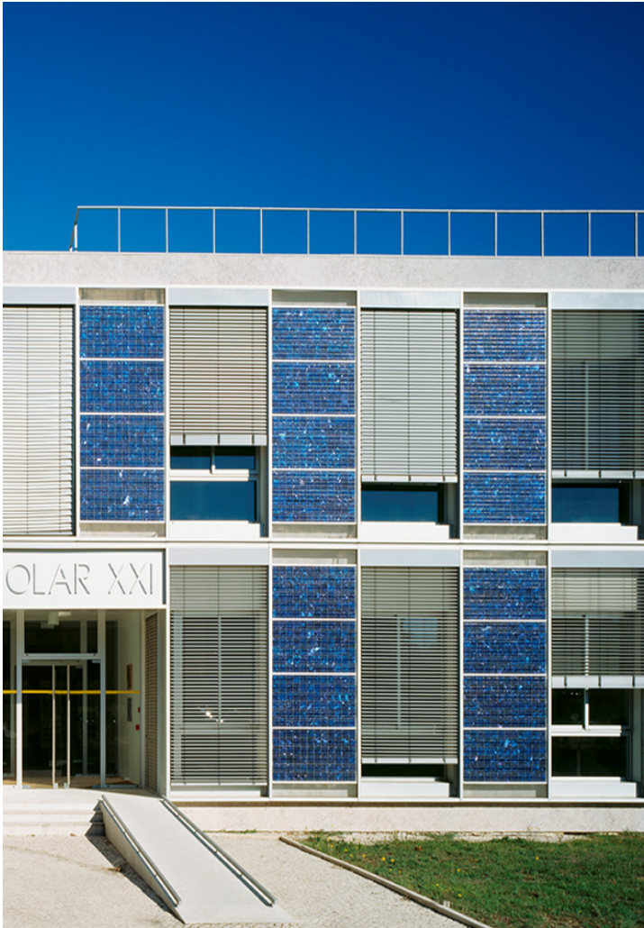
Figure 1. BIPV-T and Windows shading. BIPV-T scheme.
