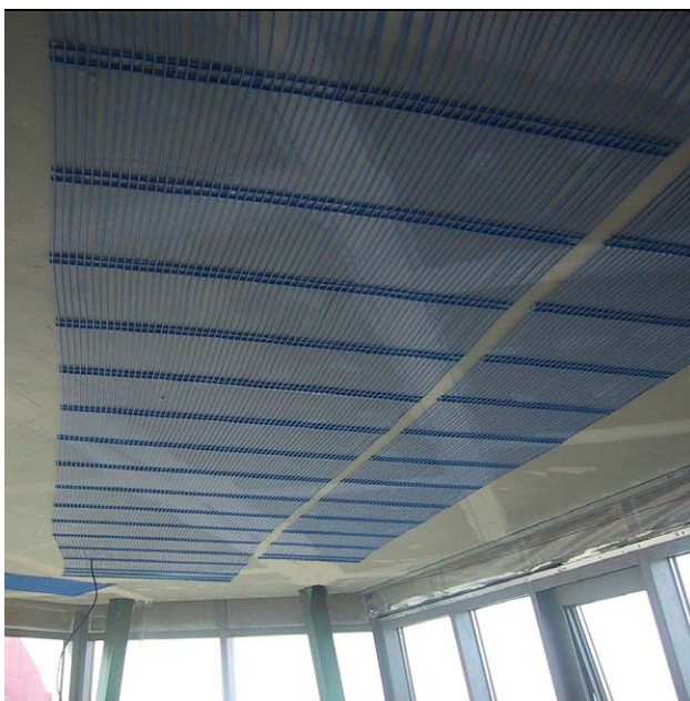
Figure 1. Integrated heating/cooling ceiling system with capillary mats before covering with the plaster.
