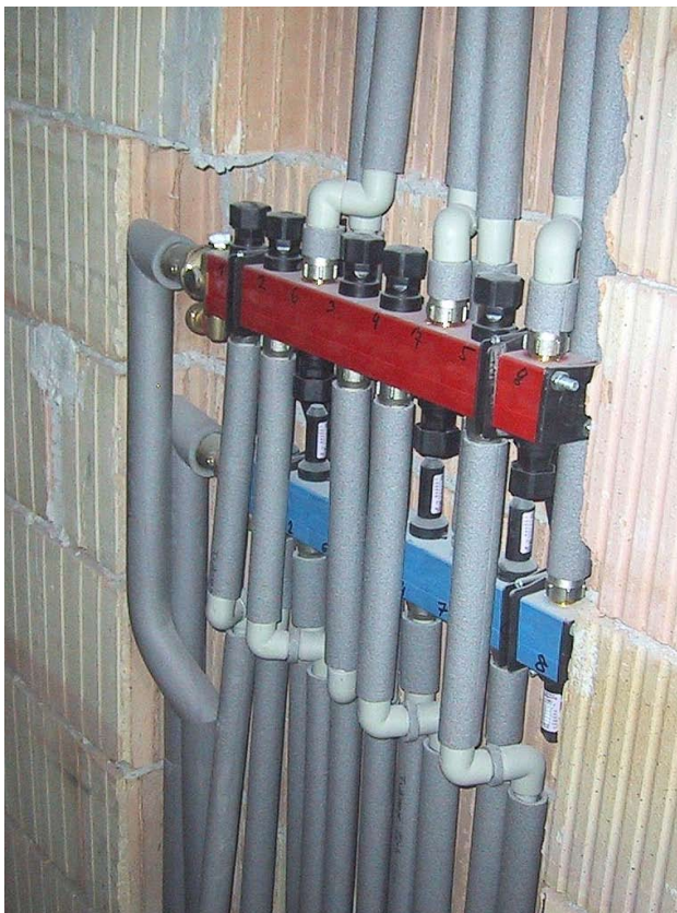
Figure 3. Four pipe system – connection circuits.
