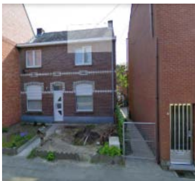
Demonstration facility 3 Belgium (mild cold) Co-ax GSHE + HP prototype n. 3
