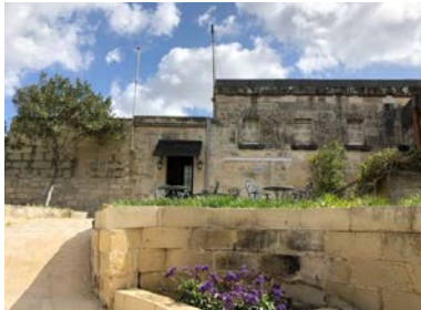
Demonstration facility 1 Malta (warm) Co-ax GSHE + HP prototype n. 1
