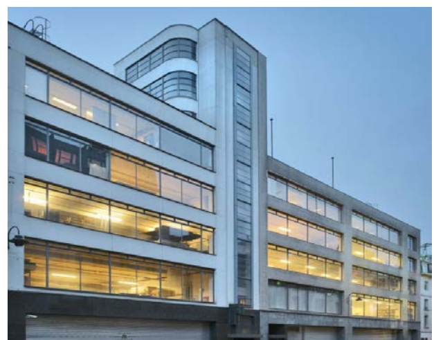
Figure 3. Technical building façade at 41 rue Fossé aux Loups.
