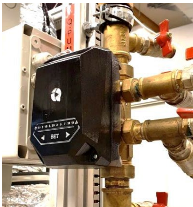
Figure 5. One-pipe control pump device: brass-casted and machined body with injection-moulded electronics cover.
