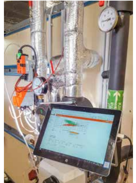
Evaluation of the recorded data to optimise delta T and the V_{max} value in the roof ventilation centre.
