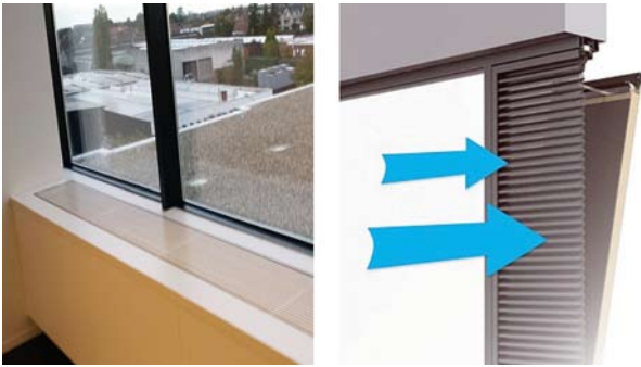
Figure 4. Supply of fresh air through skylights housed in casing.
