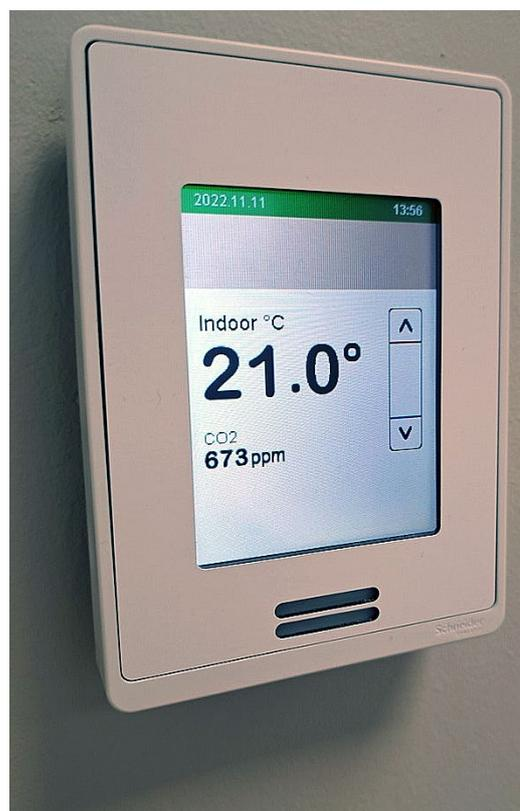
**Figure 3.** In non-residential new buildings it is expected that demand-controlled ventilation and air conditioning systems contribute to zero emission building energy performance. Temperature and CO<sub>2</sub> based control would be essential for effective ventilation and room conditioning units' operation.
