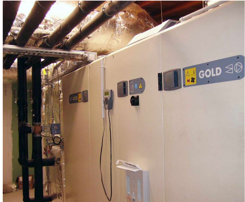
Figure 2. Chilled beam during installation. Figure 3. AHU with rotary exchanger.
