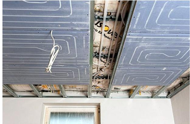
**Figure 3.** Uponor Renovis is a drywall system in which piping has been pre-installed at the factory. The elements can be mounted on virtually all wall substrates. This makes Renovis also ideal for renovation projects.
