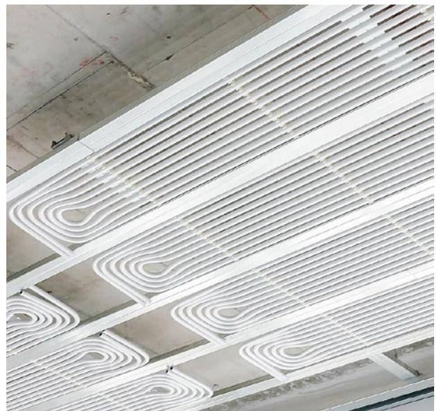
**Figure 2.** Uponor ThermoTop M is a suspended radiant heating and cooling ceiling system that consists of diffusion-resistant multilayer composite pipes. It is mounted on conventional ceiling substructures.
