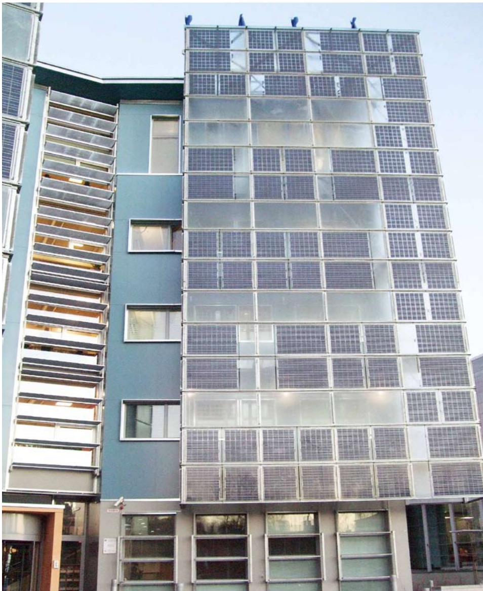
PV installation on the double facade to south serving also as an effective solar shading.
