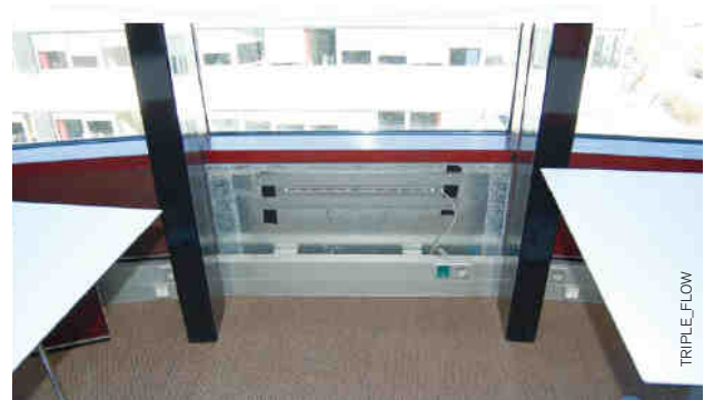
A photo of the façade intake.
