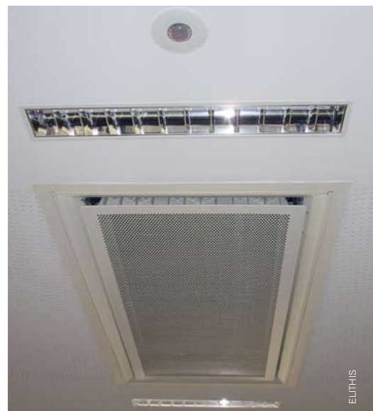
Chilled beams cassettes and lighting installation.
