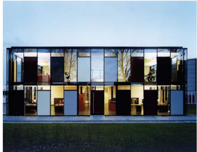
BOB (Balanced Office Building), Aachen, Germany. A highly energy efficient office building controlled by advanced building technology. Heating cooling is provided by a TAB system fed by borehole heat exchangers in combination with a heat pump.
