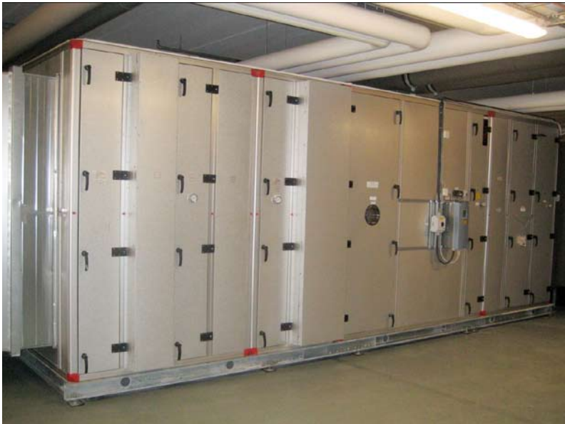
Figure 4. Low Speed Air Handling Unit without sound attenuators. The air flow is 13 m 3 /s. The speed through the AHU is 1.6 m/s.
