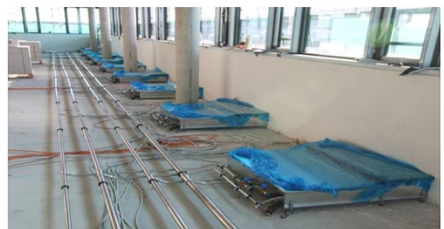
Figure 5. Application of decentralized ventilation unit; Opening in the facade (left). Decentralized devices in the room (above).
