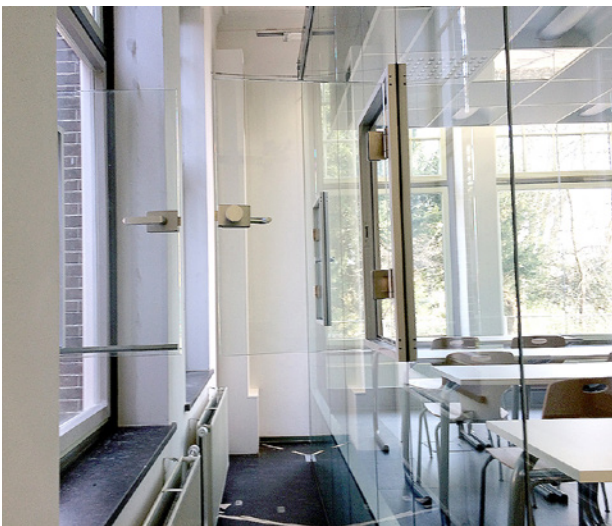
Figure 4. Operable windows and window-in-window construction in the facade.
