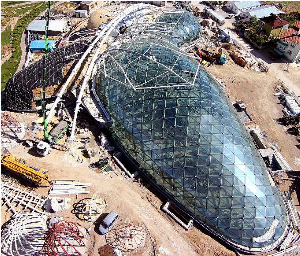
Façade details of KTBG.
