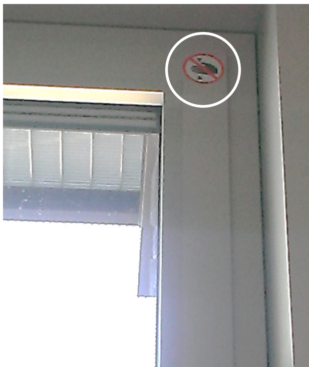
Figure 9. Ventilation flaps with additional warning pictogram and protective grid against finger injury.
