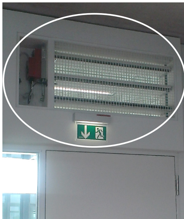
Figure 9. Ventilation flaps with additional warning pictogram and protective grid against finger injury.
