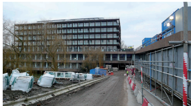
Figure 1. The Imperial Tobacco building during refurbishment (2011).
