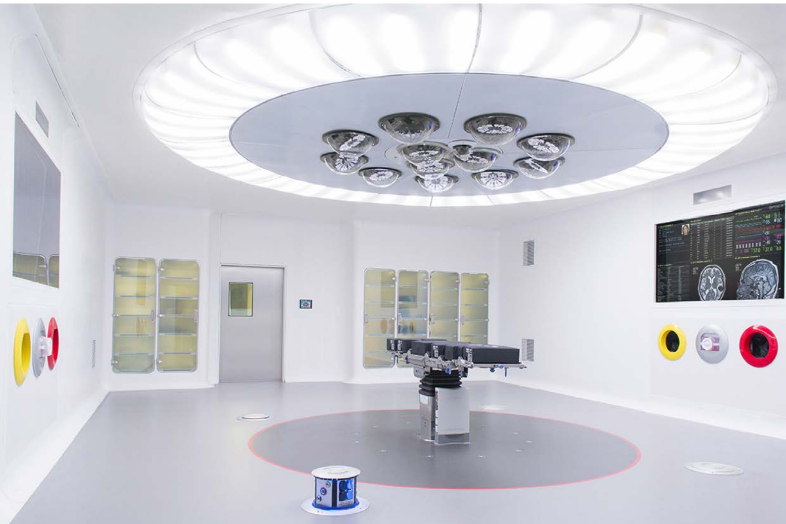
Figure 5. Optimus Integrated Surgical Environment – UDF ventilation principle [21].
