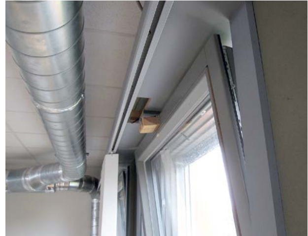
Figure 3. Principle of natural night ventilation (left) and detail of motorized window (right).
