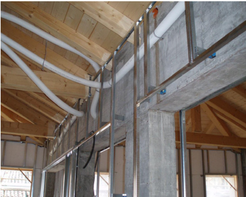
Figure 5. Mechanical ventilation system: ducts and Heat Recovery.
