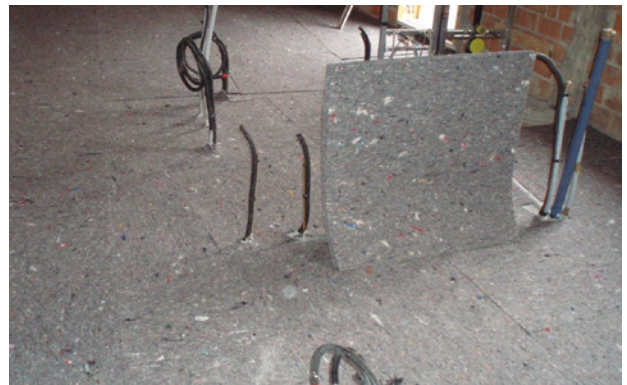
Figure 4. Radiant system: collectors (left) and TNT underflooring above system (right).
