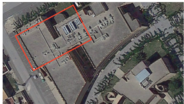
Figure 3. View from Top. HVAC Installations.
