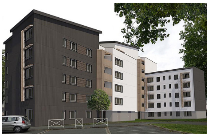
Figure 7. VLS 500 after retrofit.
