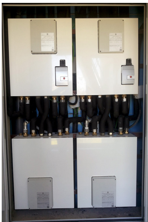
Figure 5. Energy Hubs in the technical room (top) and on each floor (bottom).
