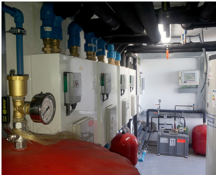
Figure 5. Energy Hubs in the technical room (top) and on each floor (bottom).
