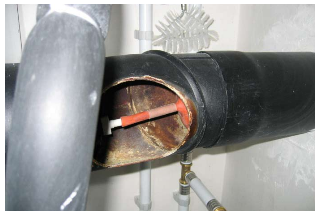
Figure 4. Access hatches in chimney flues can be very useful if the flues need to be sealed for the airtightness test.
