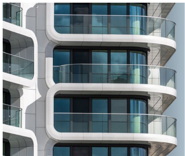
Throughout the Grand Tower, residents can adjust the room temperatures of their apartments to meet their individual needs.
