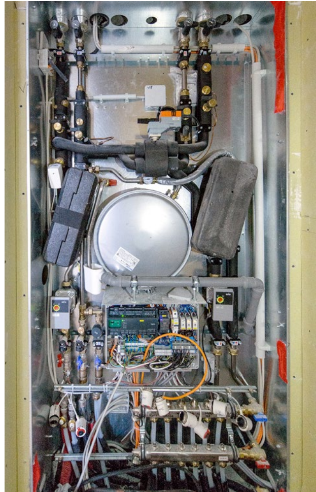
The Uponor heat interface units were specially designed for the Grand Tower project. They serve as transfer points for heat and cold to the living areas and include integrated six-way ball valves.
