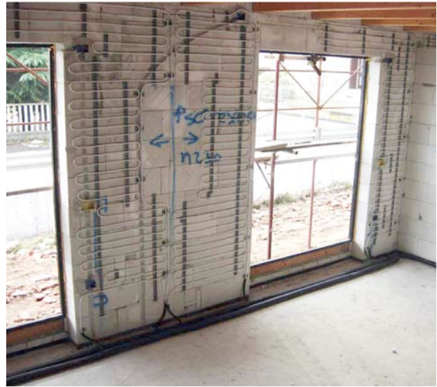
Figure 5. Installation of wall radiant panels.
