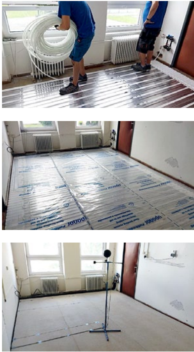
Figure 2. Floorplan of the room 202.1 with radiant floor system and placement of sensors. (Author: Martin Šimko, Uponor, s.r.o.)
