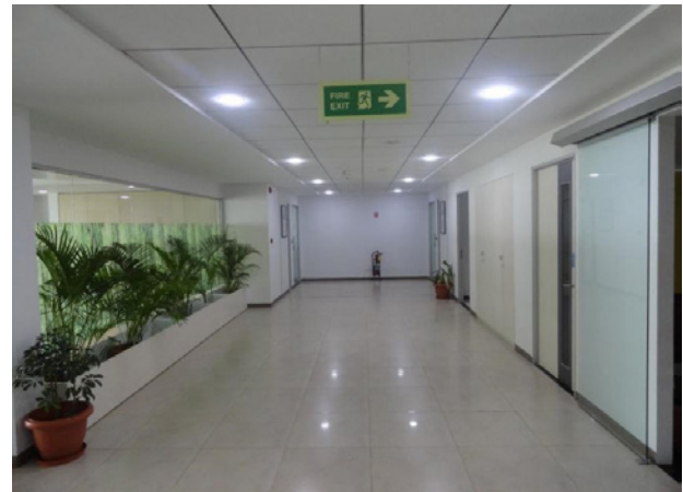
Efficient LED lighting in the building.
