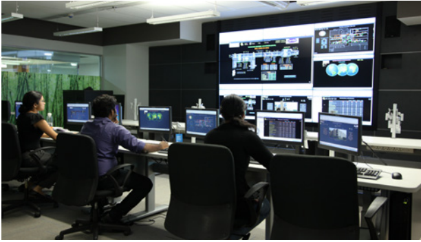
Central Command Center for monitoring performance.
