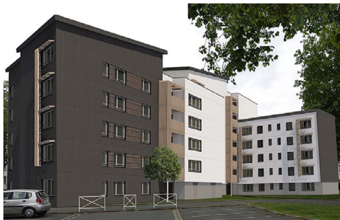
Figure 7. VLS 500 after retrofit.
