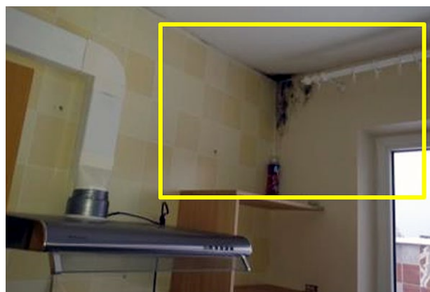
Figure 1. Example of light renovation with deteriorated IAQ. Replaced, new airtight window has blocked ventilation resulting in mould growth on thermal bridges. Thermal image on the left, photo on the right.
