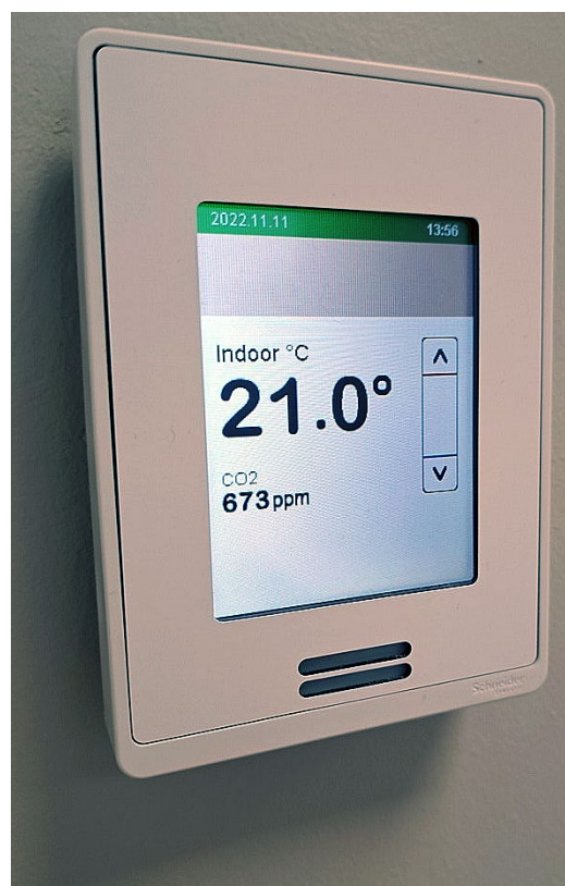
Figure 3. In non-residential new buildings it is expected that demand-controlled ventilation and air conditioning systems contribute to zero emission building energy performance. Temperature and CO 2 based control would be essential for effective ventilation and room conditioning units' operation.
