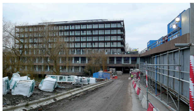
Figure 1. The Imperial Tobacco building during refurbishment (2011).
