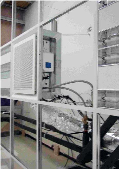
Figure 2. Chilled beam during installation. Figure 3. AHU with rotary exchanger.
