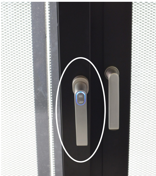
Figure 8. Automated window, with optional manual operation and resistance sensitive gasket.
