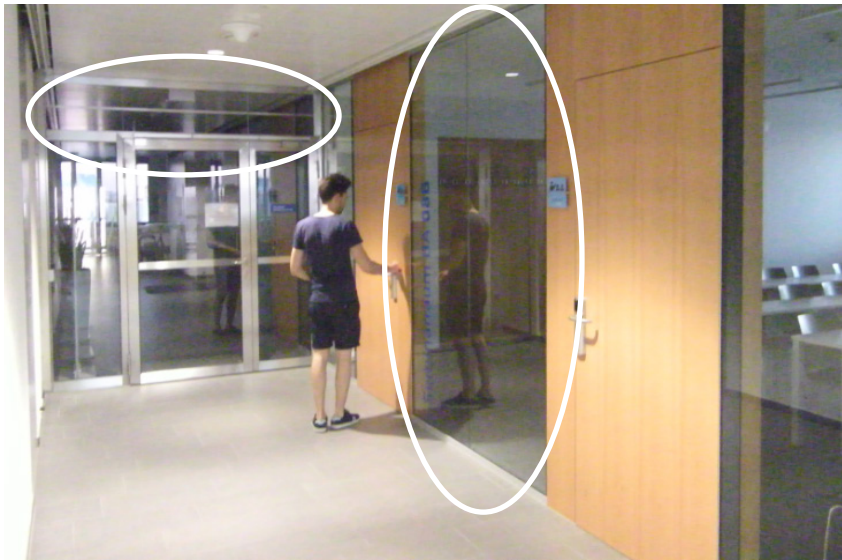
Figure 5. Glazed partition walls with high U-values and overflow orifice.
