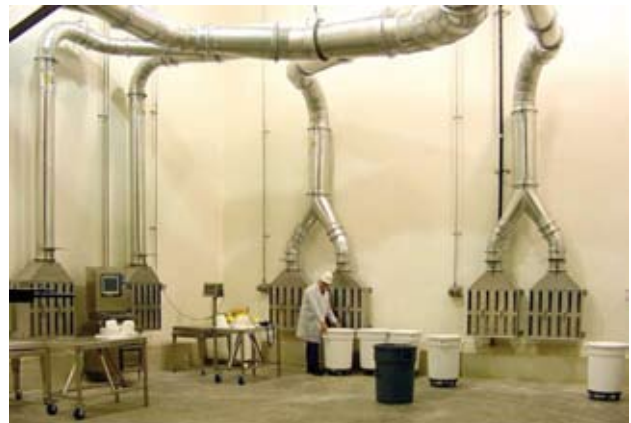
Figure 1. Typical hood system.
