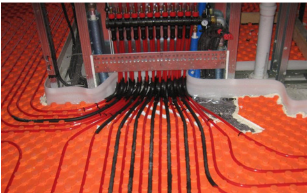
Figure 4. Radiant system: collectors (left) and TNT underflooring above system (right).
