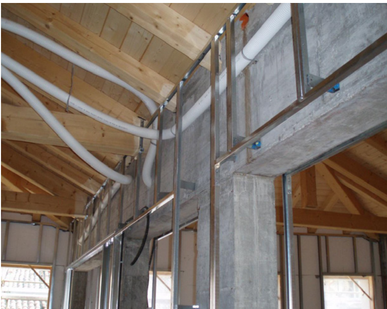
Figure 5. Mechanical ventilation system: ducts and Heat Recovery.
