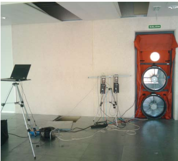
Zone sealing for airtightness testing (two first ones) and bottom one BlowerDoor installation for tightness testing
